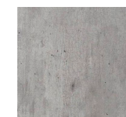
Grey Shuttered Concrete
